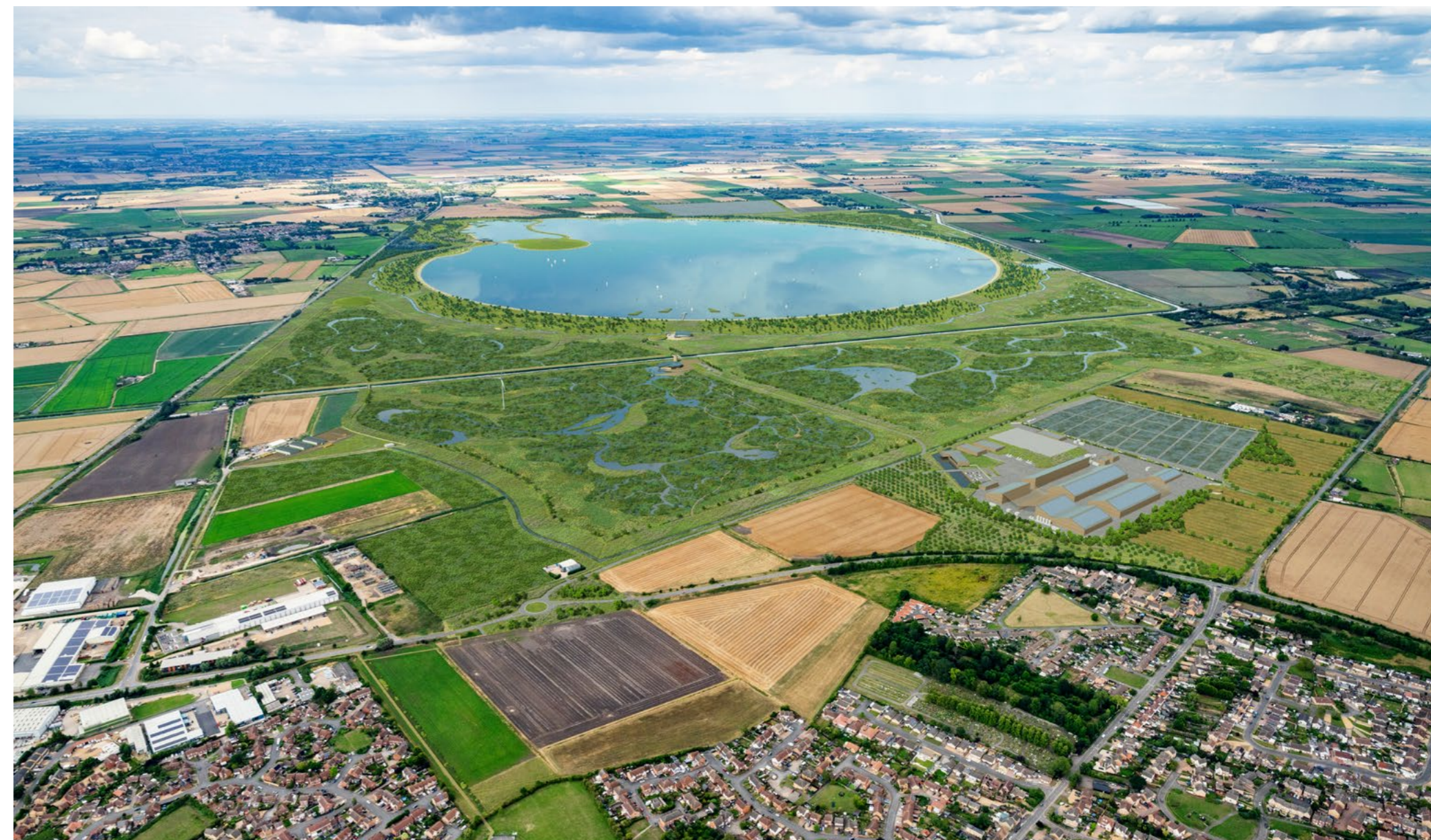
Aerial view from Chatteris, showing the A142 running along the southern boundary of the main reservoir site, and the A141 at the site's western boundary. For illustrative purposes only.
