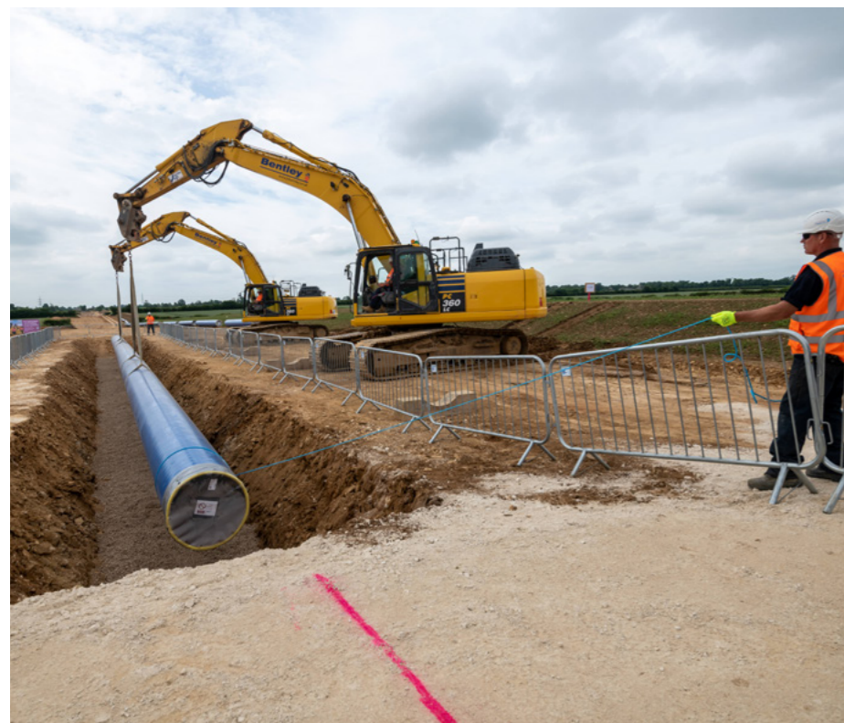
Image showing the construction of our Strategic Pipeline Alliance project.
