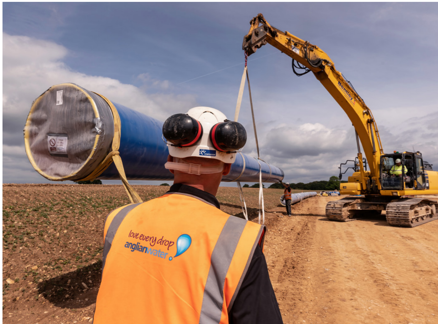
Image showing the construction of our Strategic Pipeline Alliance project.
